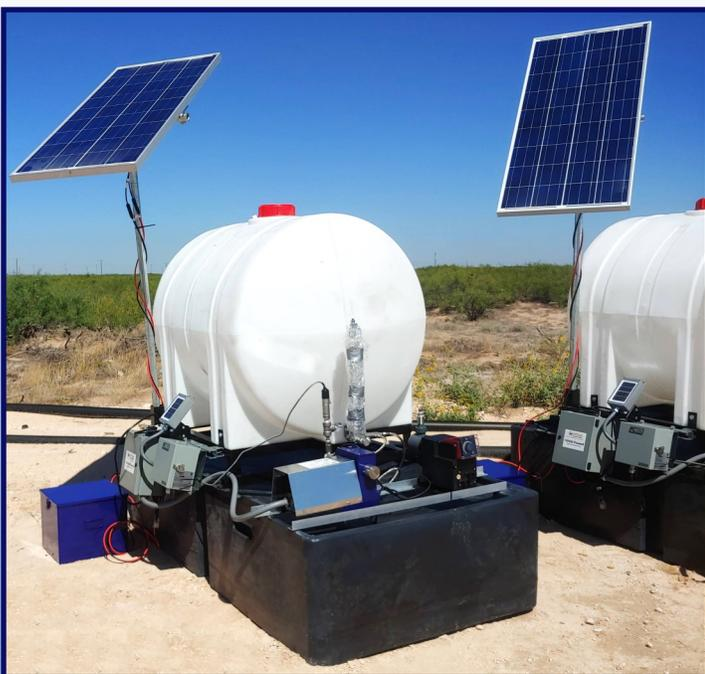
*Megas Solar Pump set up on skid*
